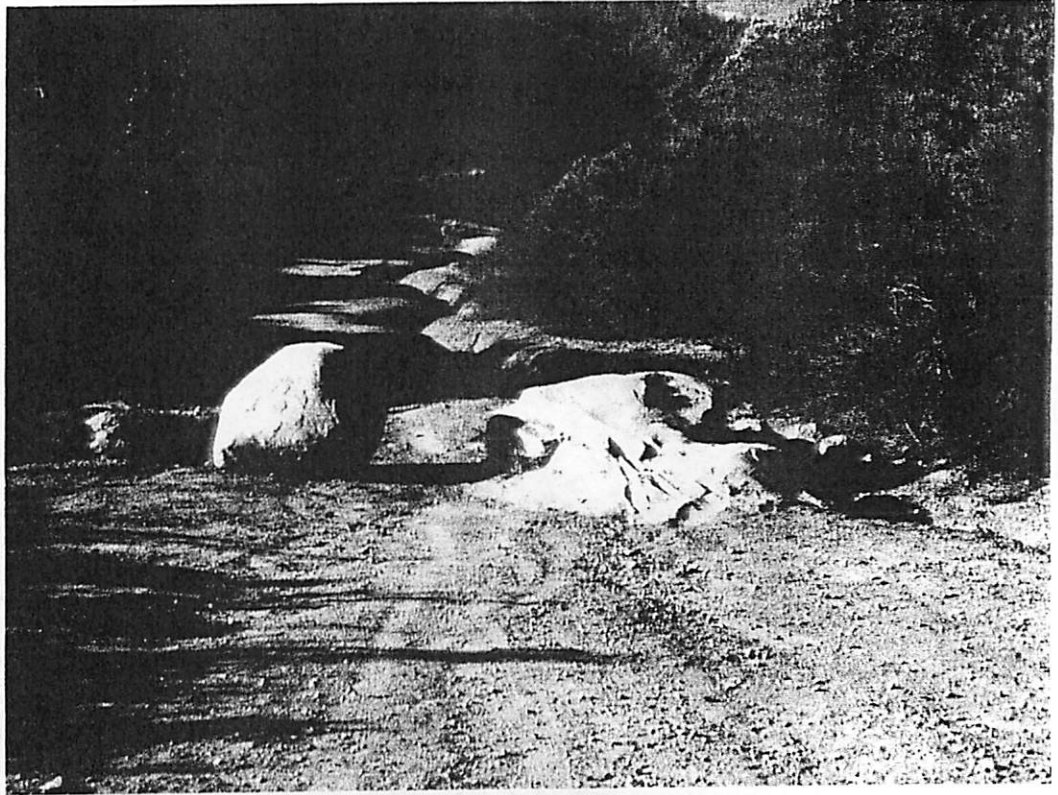
Photo 20.—Trail erosion has been a problem in the SRA.
